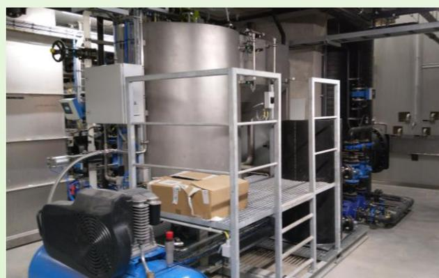
Struvite precipitation, Ghent. Image by CEIP/DuCoop
